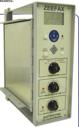
Seizing the opportunity to rectify some of the shortcomings of the original design and incorporate features which would be found on a modern generator control module, **Zeefax** opted for a digitally controlled approach for better reliability, easier configuration, improved diagnostics and enhanced functionality.
