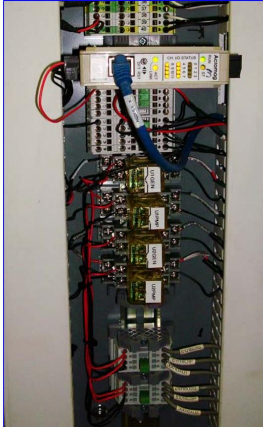
*Fig 13: Key Phase Input Control Relays*
