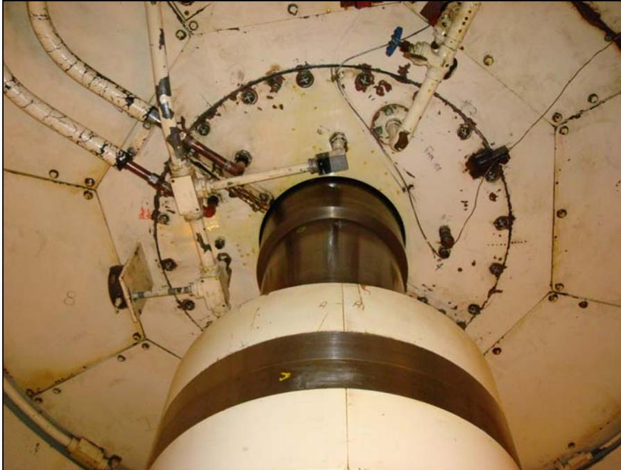
Fig 7: Lower guide bearing as found
