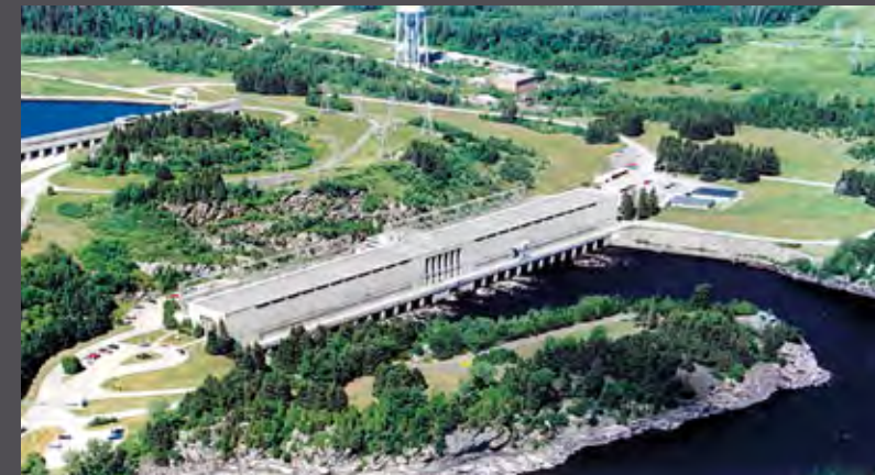
Shipshaw HPP (courtesy of Alcan Canada)
